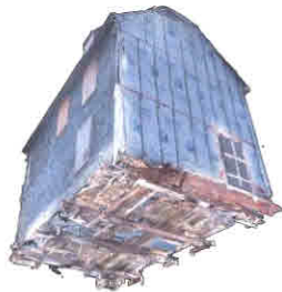
Underside and north wall
